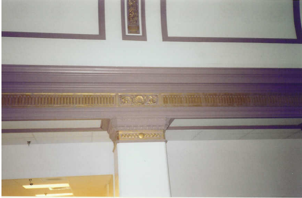
Second Floor of Main Entrance to Royce Hall
